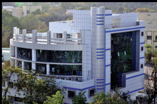
Chips Data Centre, Raipur
